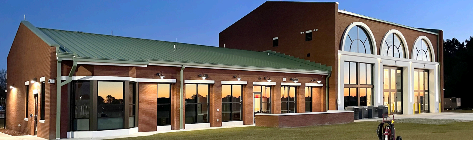
Coastal Carolina Regional Airport in New Bern opened a $5.8 million aircraft rescue and firefighting facility in 2021.
