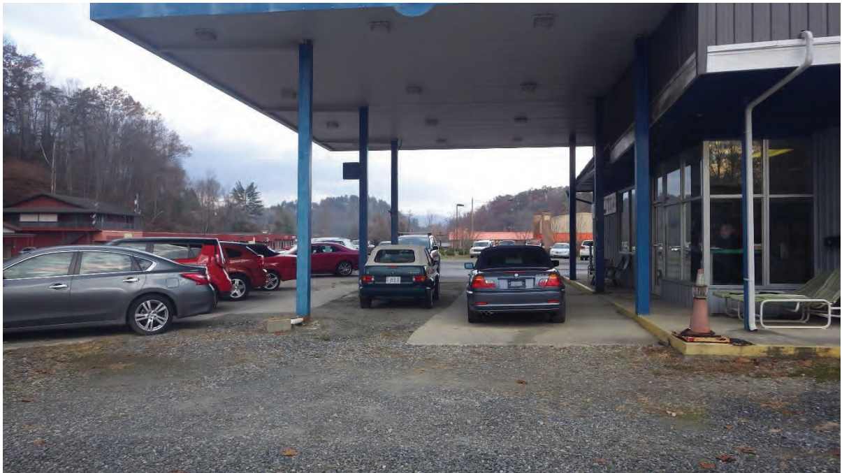
Land disturbance for USTs removal
