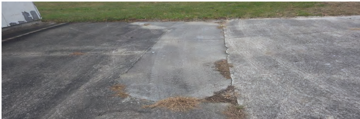
Pump island removed
