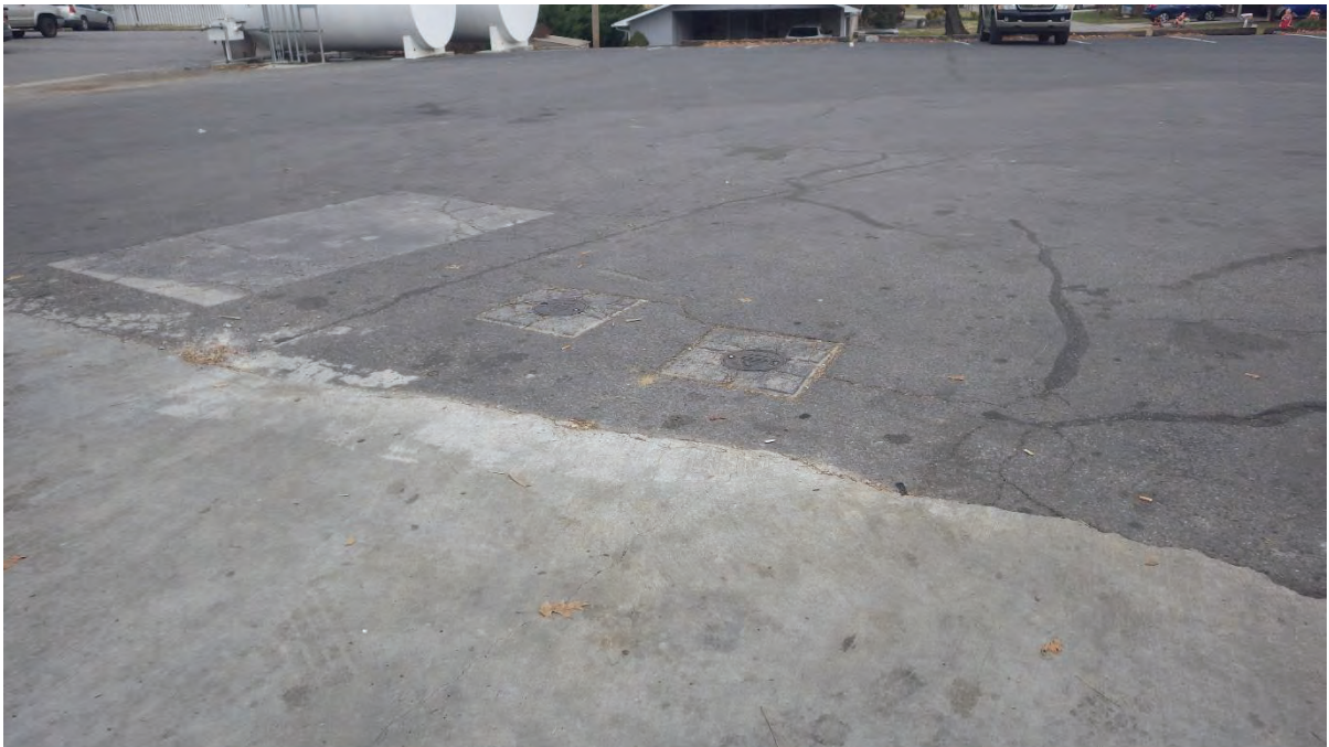
Monitoring wells in pairs.
