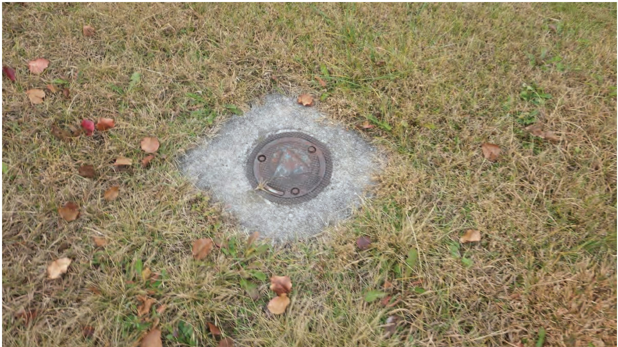
Older Monitoring well
