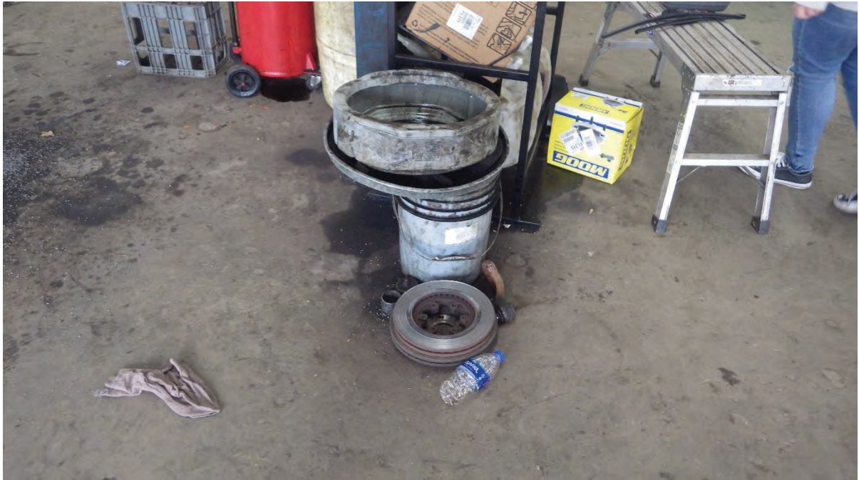
UST fill port inside the building according to an employee on site.
