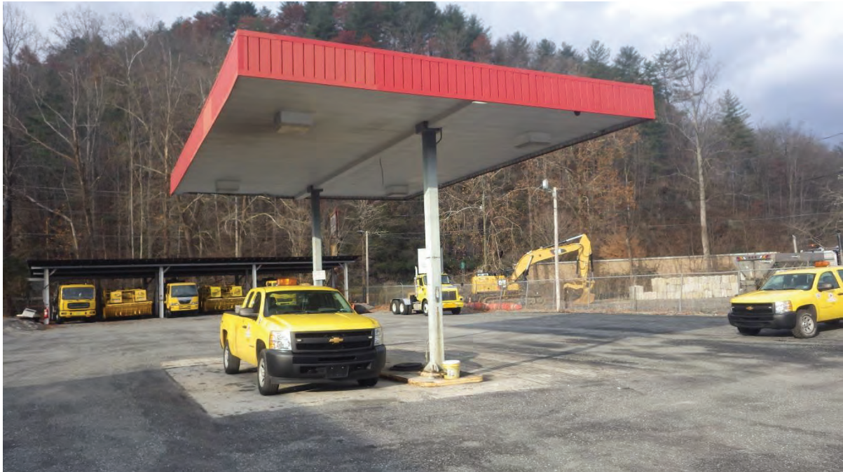
Former dispensers area
