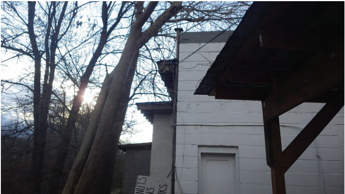
Two vent pipes on the wall.
