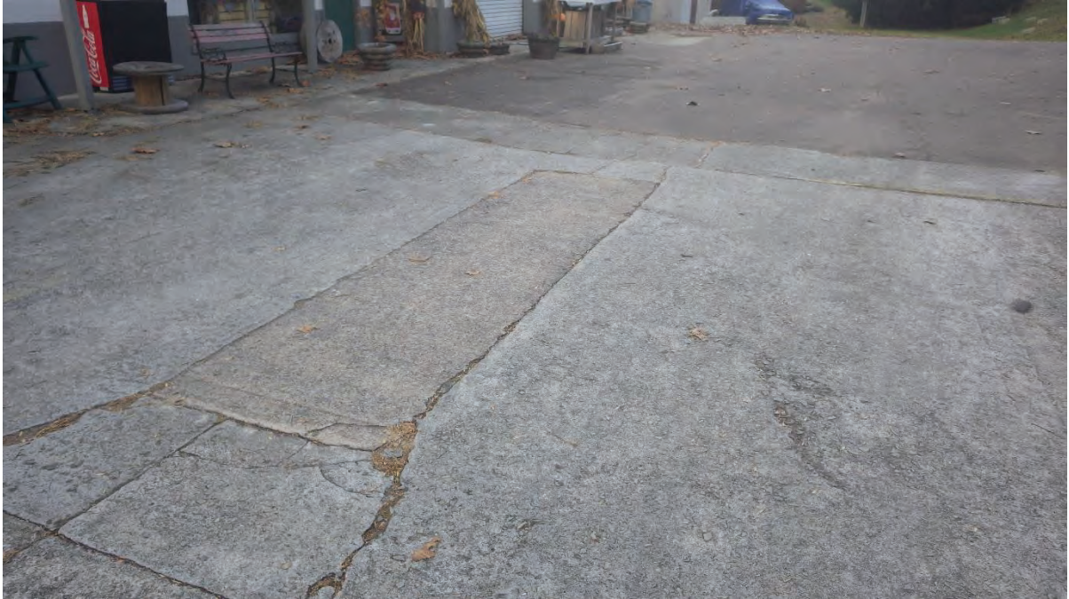
Former dispenser area
