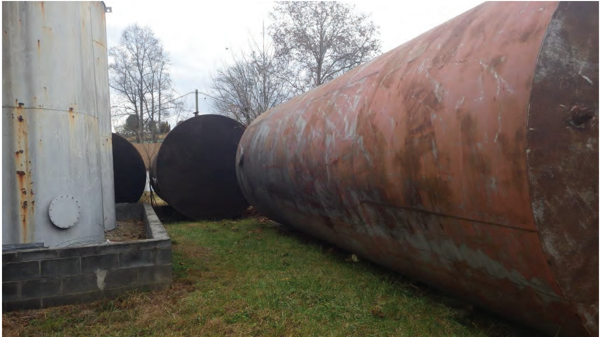
Some USTs removed and store on site.
