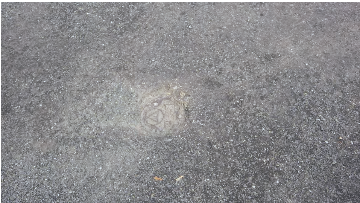
Monitoring well in the former USTs area
