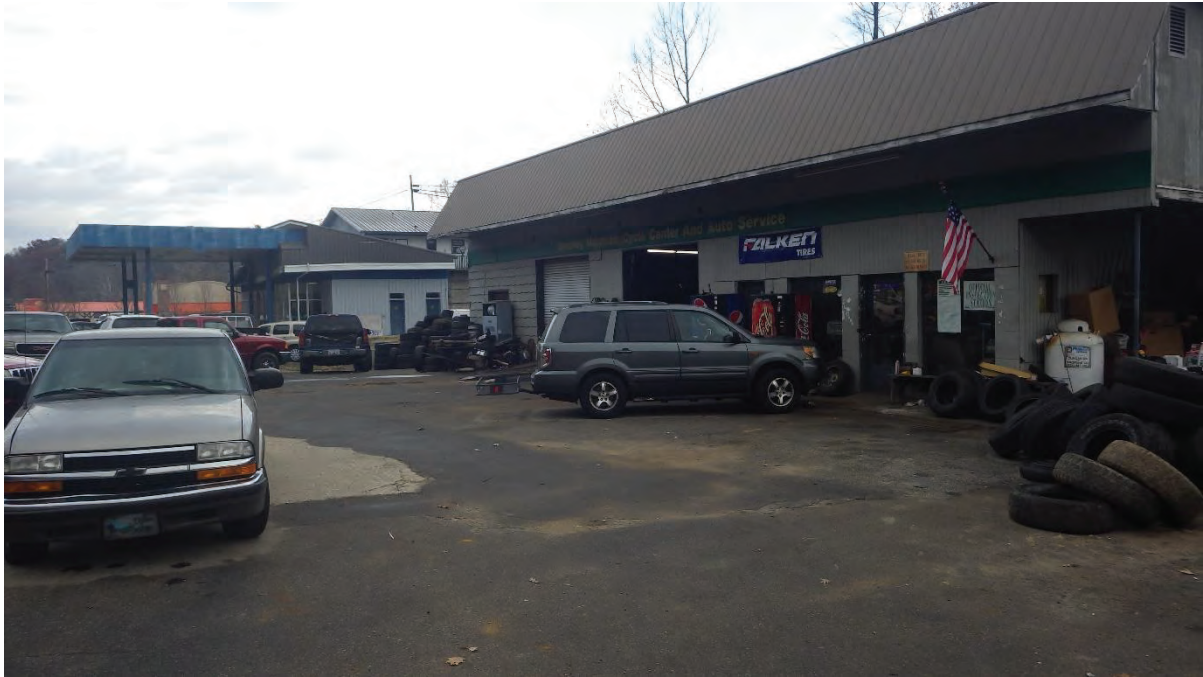
Pavement disturbance appears to be for UST removal
