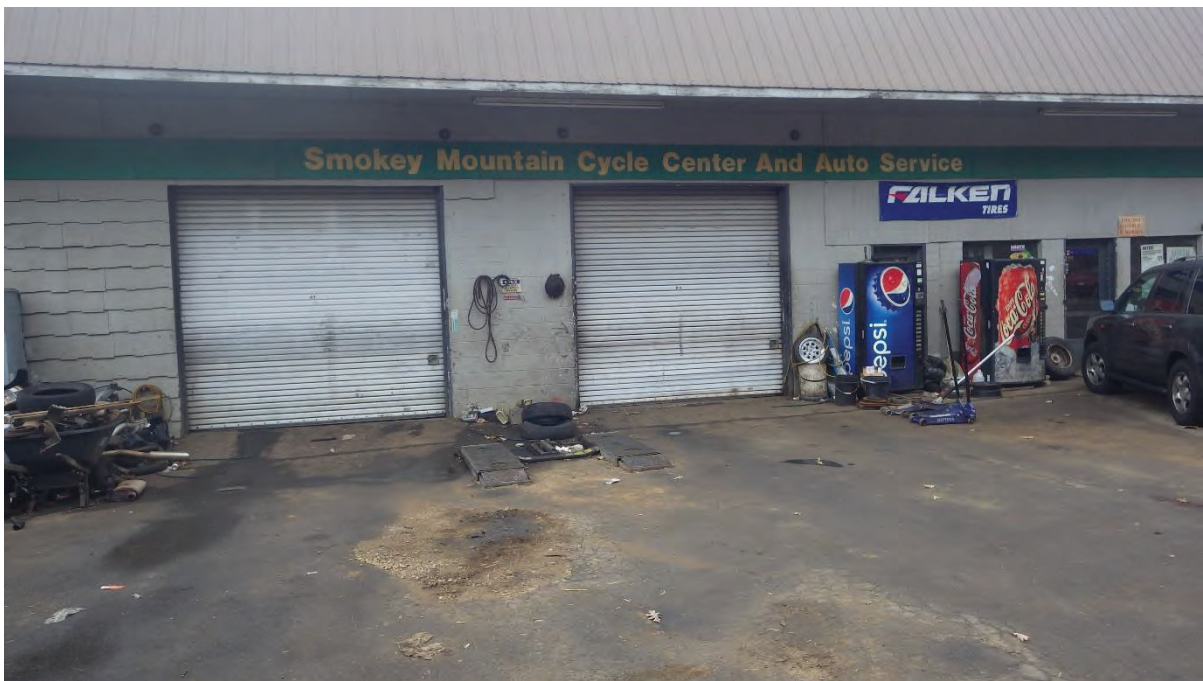
Two bays with in-ground hydraulic lifts.
