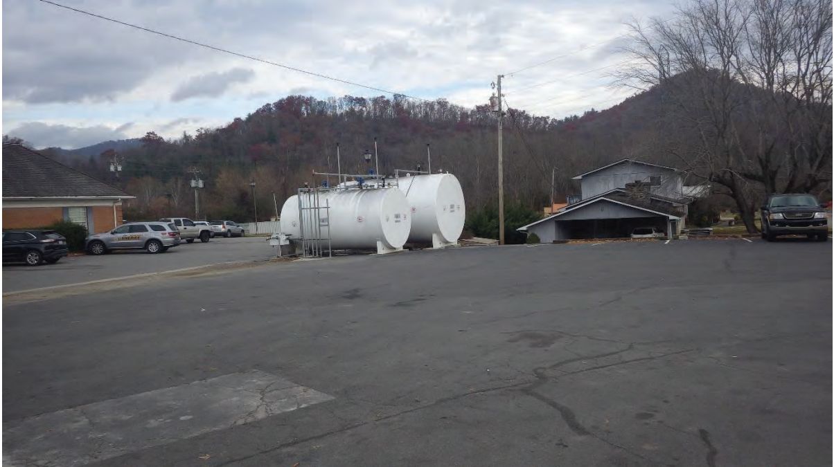
ASTs with concrete internal lining.
