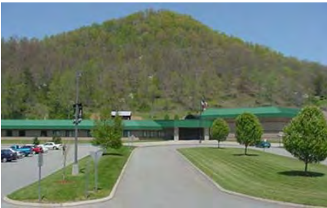
Figure 3: Robbinsville High and Middle School building
