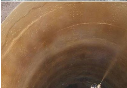
Installation of SprayWall® on steel pipe (Top), Installation of SprayWall® on concrete pipe (Bottom) – images from SprayROQ™ website
