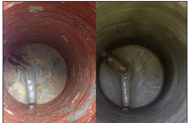
Before (left image) and after (right image) example of Quadex® Qm-1s Restore applied to a vertical shaft originally constructed of brick – image from Vortex technical data sheet
