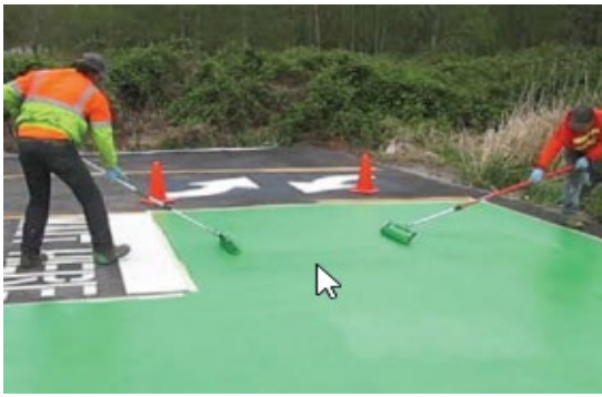
Image of Vanguard EcoPath Coating being applied (Left) and a completed bicycle path marking (Right). Images from Vanguard’s website.
