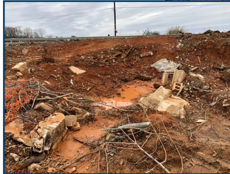
Winston-Salem Northern Beltway (Forsyth County)
