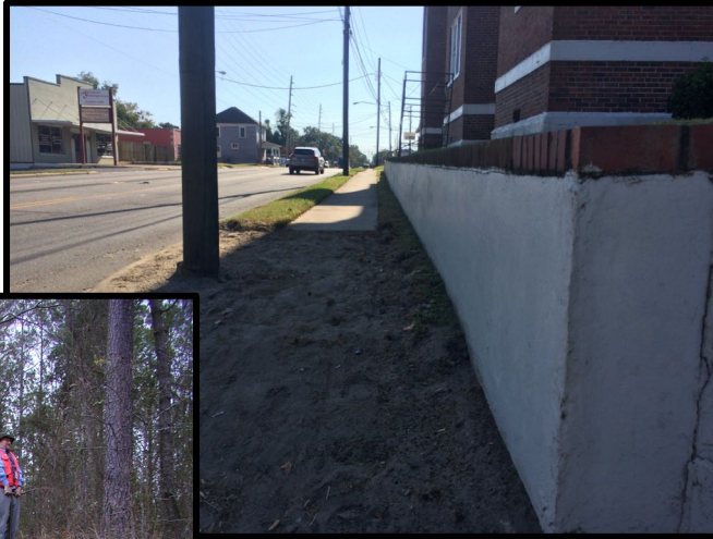
Respass Street Remains Recovered during Sidewalk Installation (Beaufort County)
