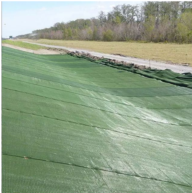
Image of TRM-270 installed on a slope from NCIF's website.
