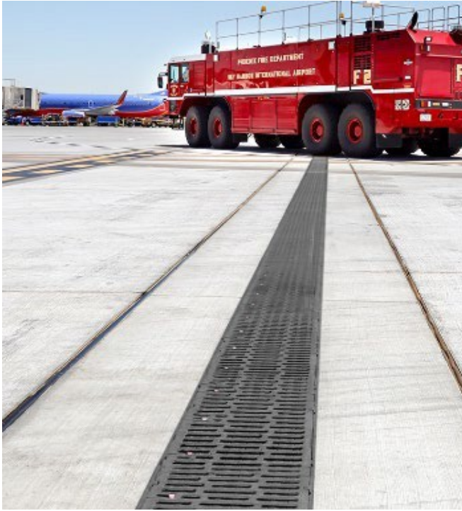
Image of ACO PowerDrain® installed on an airport runway (left) and a generated image of a single section (right) from ACO's website.
