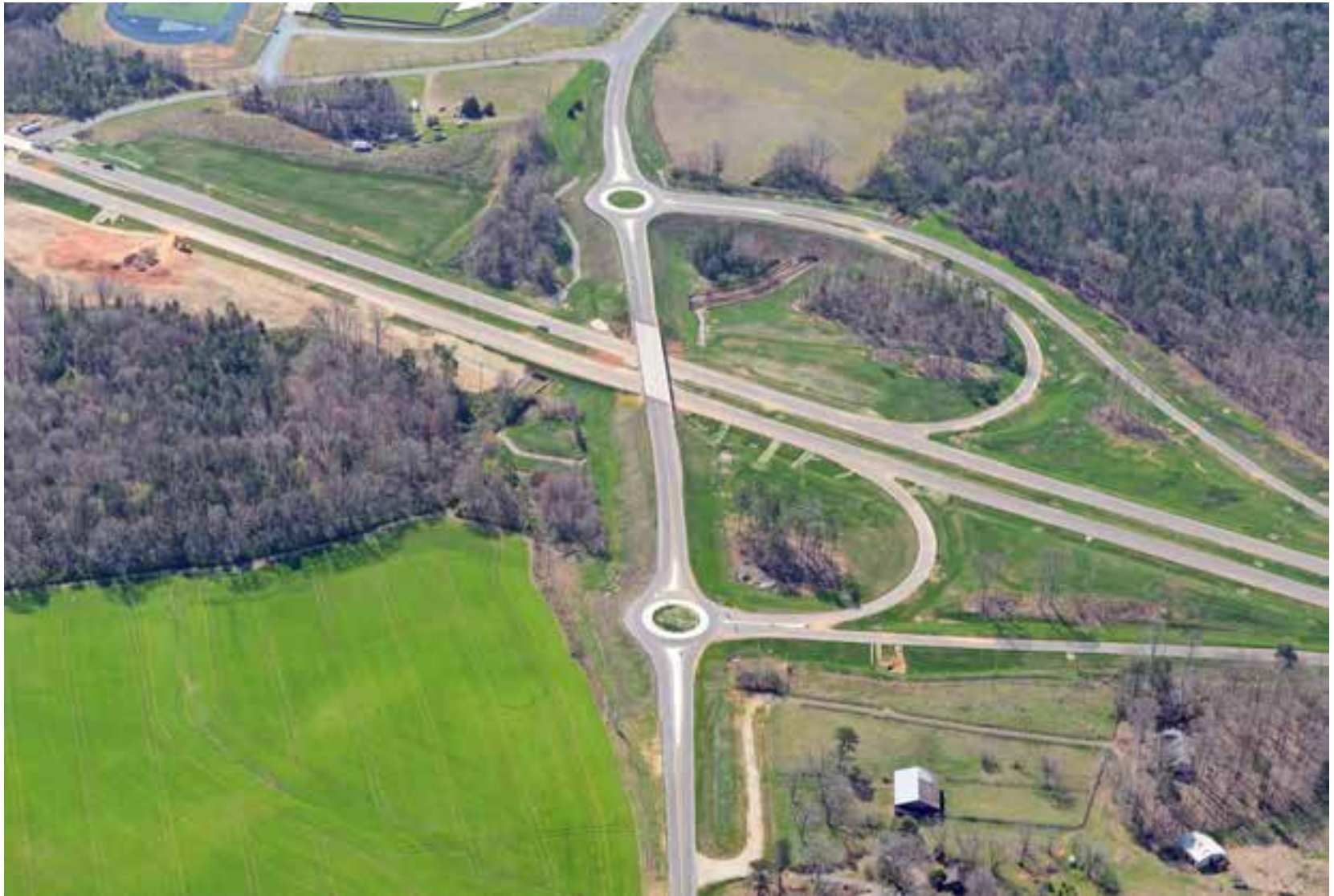
Austin Chaney Road Interchange
