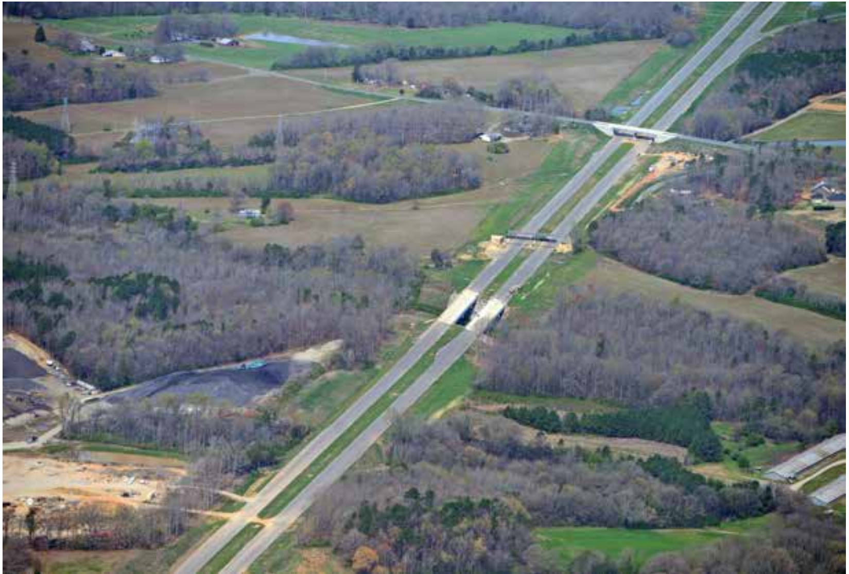
Toll Zone 6 Between US 601 and Morgan Mill Road
