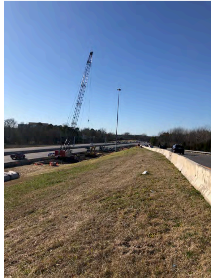
Johnston Road Direct Connect Bridge
