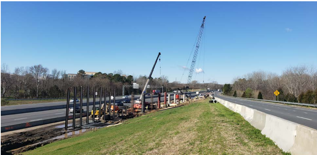
Johnston Road Direct Connect Bridge
