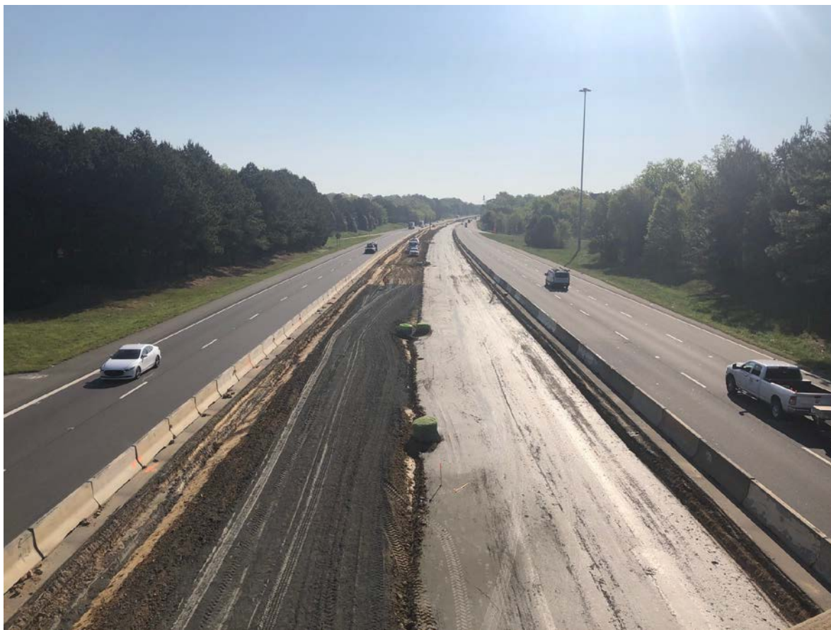
Segment C soil stabilization
