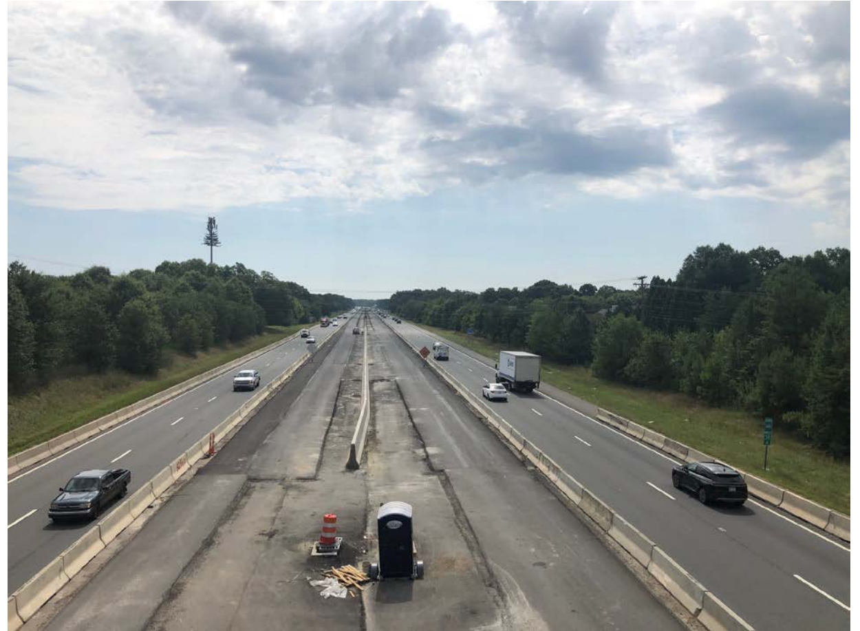
Segment C Median Widening near Ballantyne Commons Parkway
