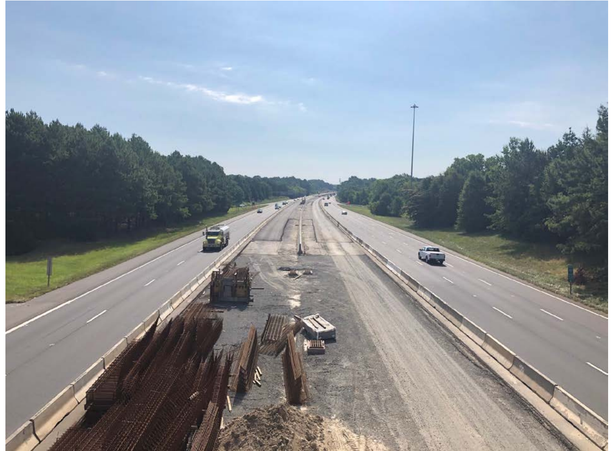
Segment C Median Widening near Rea Road
