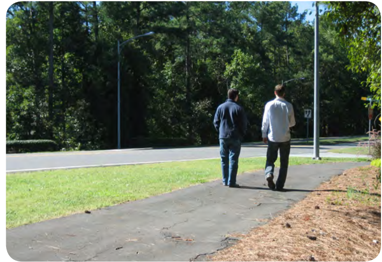
Sidewalk without curb and gutter in Durham, NC.
