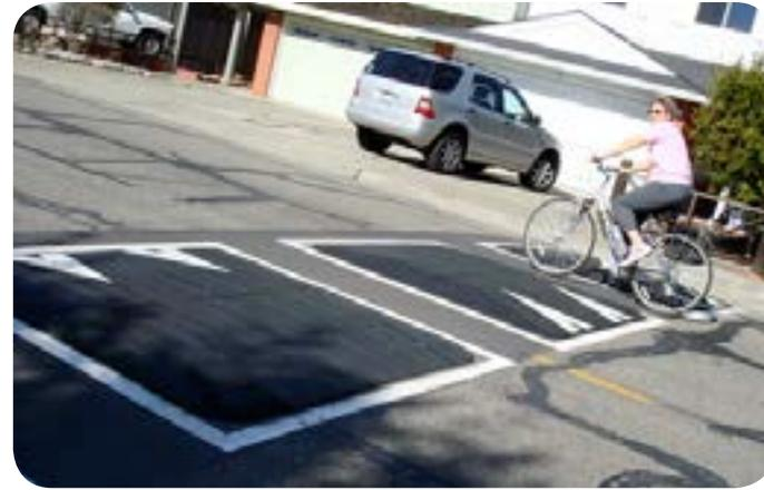
**Road Diet for decreased crossing distance:** Roadway narrowing can improve conditions and safety for pedestrians by decreasing vehicle speeds and the distance pedestrians have to travel to cross the street. Roadway narrowing can be achieved by narrowing vehicle lanes, removing travel lanes, adding on-street parking, or other means.
