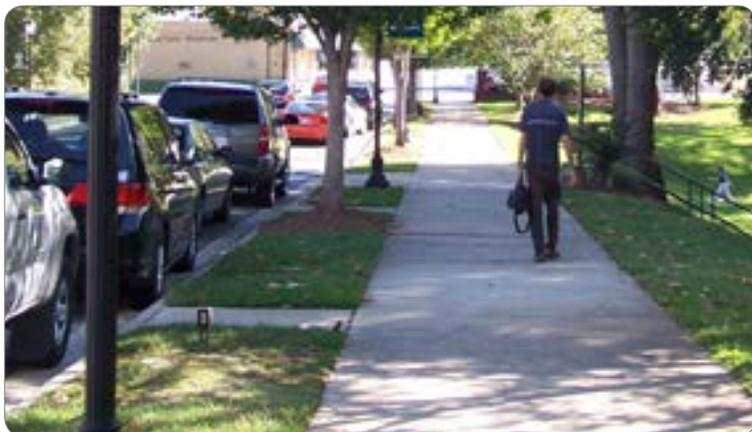
A buffer zone is a strip of land that separates vehicular traffic from the sidewalk or other pedestrian facility. A pedestrian's safety and comfort in the roadway environment is significantly affected by the width and quality of the buffer between the sidewalk and the roadway, especially on streets with heavy traffic volumes. A minimum buffer zone of six to eight feet is desirable, and will vary with the street type and surrounding land uses.
