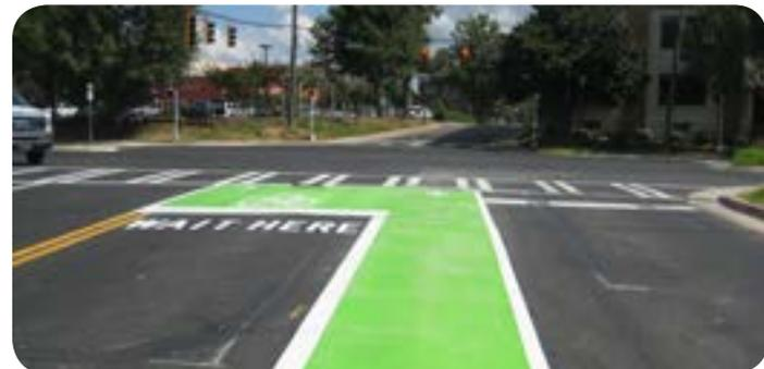
**Right Turn Through Bike Lane:** Right-turn-only lanes are often used where right-turning motor vehicle volumes warrant an exclusive right-turn lane to improve traffic flow. The correct placement of a bike lane is on the left of an exclusive right-turn lane. Incorporating the bike lane to the left of the right-turn-only lane enables bicyclists and right turning motorists to sort their paths by destination in advance of the intersection, avoiding last moment conflicts. (AASHTO)
