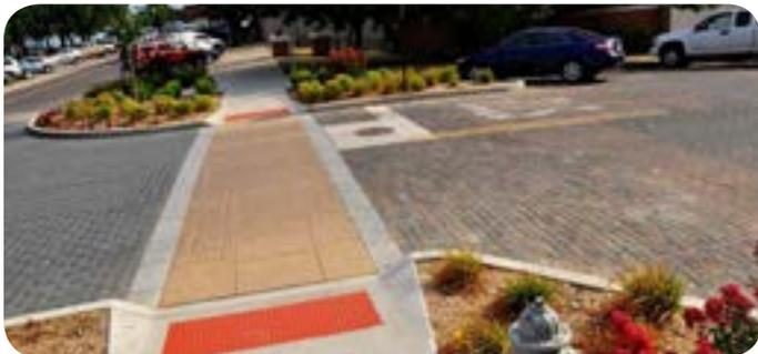
**High visibility crosswalks:** High visibility crosswalks use specific marking patterns to increase the visibility of the crosswalk to approaching motorists. Traditional crosswalks have two lines perpendicular to the direction of motorist travel, and are often difficult for motorists to see. High visibility crosswalks use wider lines perpendicular to traffic, but also add wide lines parallel to the direction of motorist travel, which greatly increases the visibility of the crosswalk.
