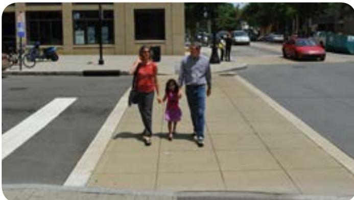
**Curb Extensions:** Curb extensions (also called bulb-outs or bump-outs) are extensions of sidewalks that narrow the street, increase pedestrian visibility, and decrease pedestrian crossing distance. They are an element of traffic calming that prioritizes pedestrian safety, reduces vehicle speeds, and serves to protect on-street parking. Curb extensions should however not intrude into a bicycle lane.
