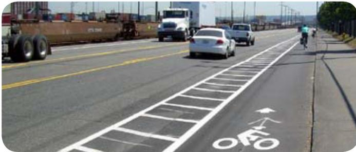
**Contra-Flow Bike Lane:** Contra-flow bicycle lanes are bicycle lanes designed to allow bicyclists to ride in the opposite direction of motor vehicle traffic. They convert a one-way traffic street into a two-way street: one direction for motor vehicles and bikes, and the other for bikes only. Contra-flow lanes are separated with yellow center lane striping. (NACTO)
