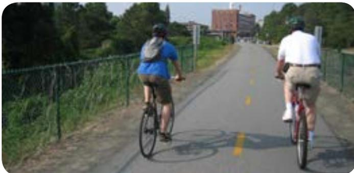
**Sidepath:** Sidepaths are multi-use paths that are located exclusively adjacent to a roadway, typically within the road right of way. These provide space for bicycle and pedestrian travel where on-road bicycle facilities are not feasible due to traffic volumes, speeds, or roadway configuration (such as limited access highways, for example).
