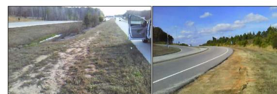
**Figure 4: Turf Failures**
