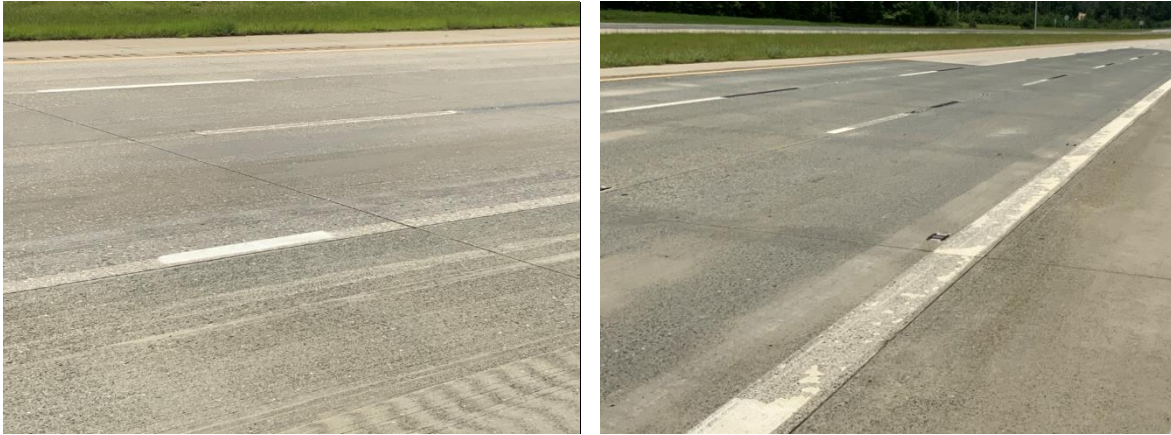
Figure 3: Pavement Striping Inspection Results Sample
