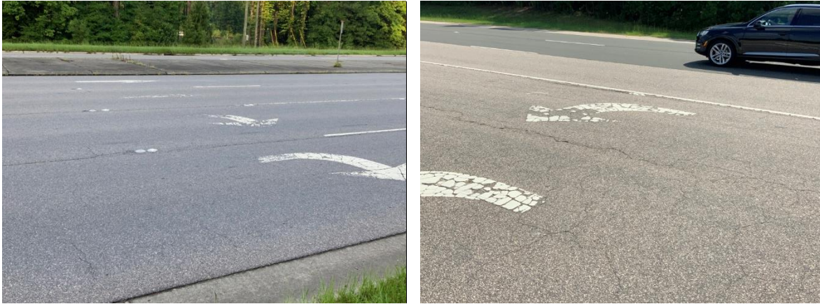
Figure 4: Pavement Symbol Inspection Results Sample
