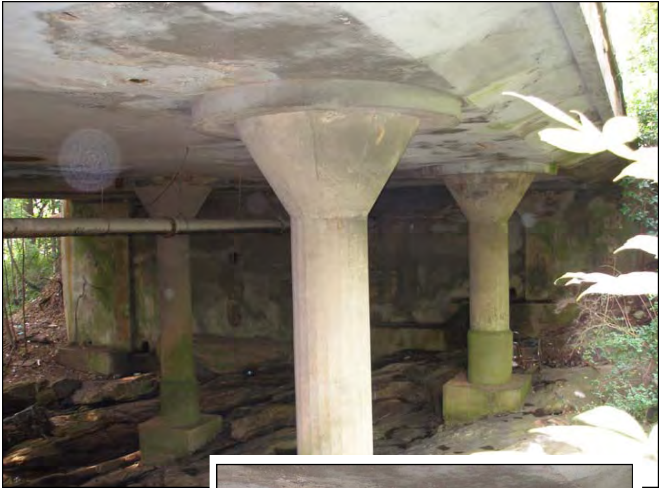
Cameron Avenue Across Falling Branch Mushroom Column Design Built: 1920
