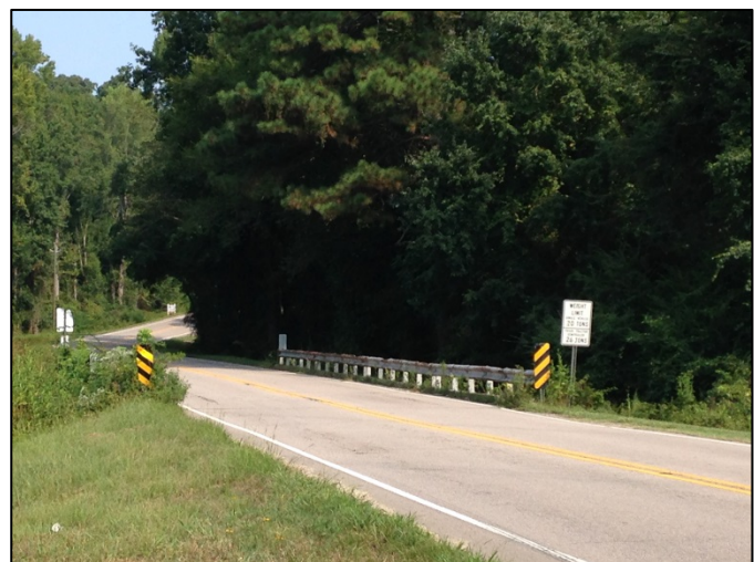
Looking Northeast Towards Bridge No. 126
