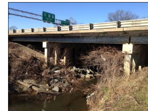
Existing Bridge No. 299
