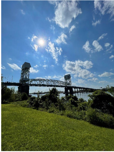
Figure 1: Cape Fear Memorial Bridge (view East-West)
