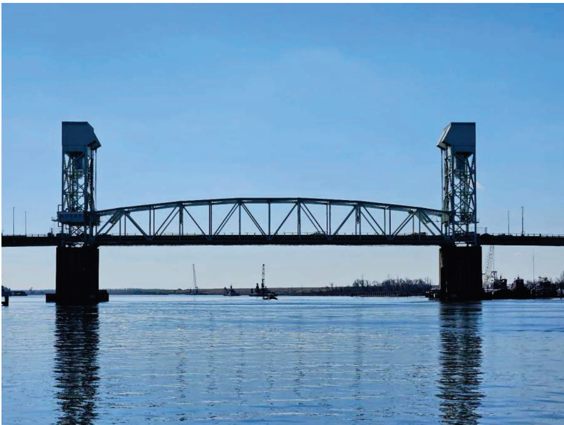
Figure 5: Cape Fear Memorial Bridge Looking Downstream
