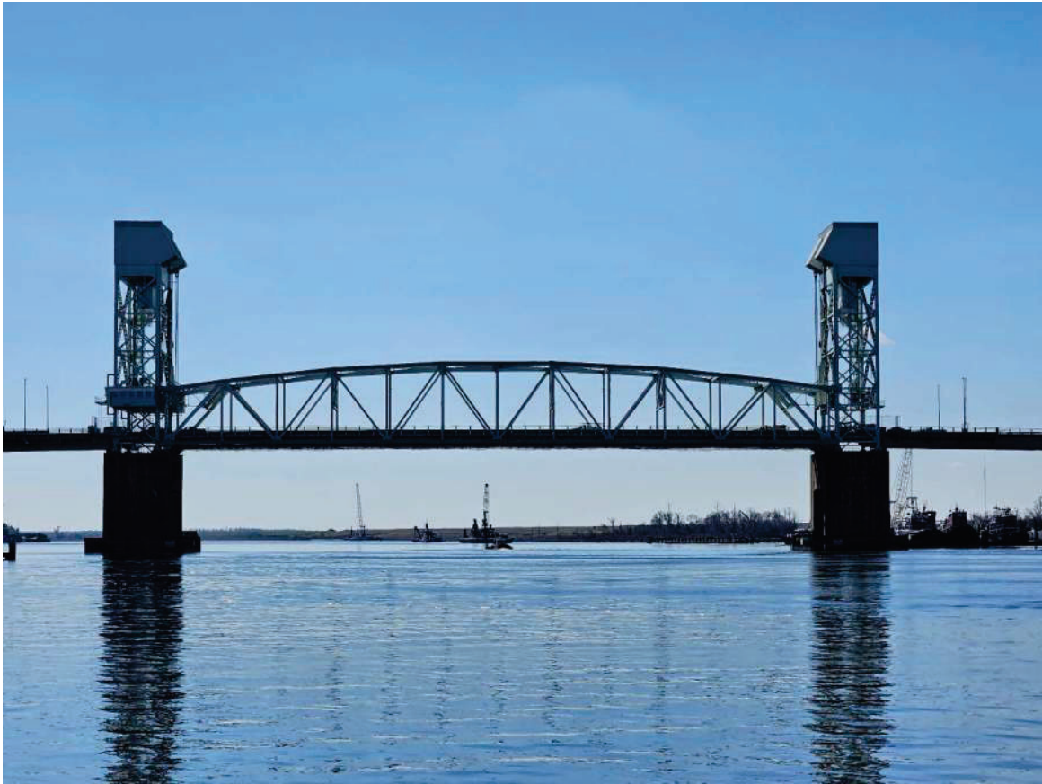
Figure 1: Cape Fear Memorial Bridge Looking Downstream
