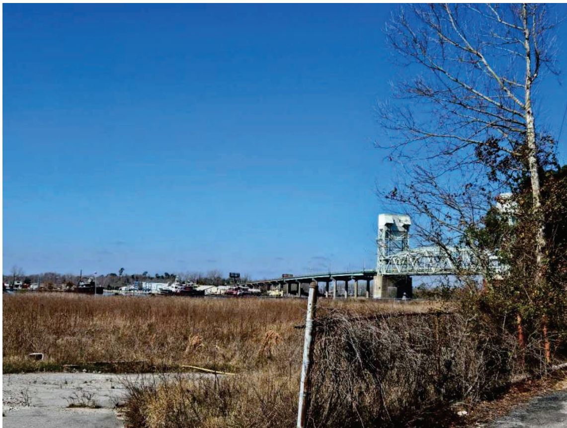
Figure 6: Downstream of Cape Fear Memorial Bridge Looking West.
