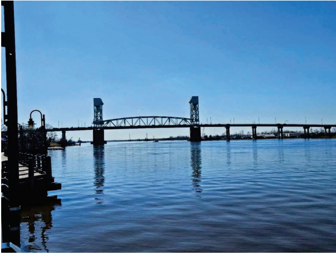
Figure 2: Cape Fear Memorial Bridge Looking Downstream from Wilmington Downtown Riverwalk.
