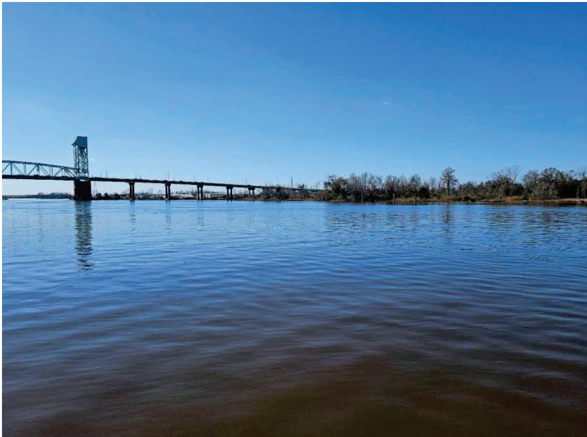
Figure 3: Cape Fear Memorial Bridge Looking Downstream Towards West Bank from Wilmington Downtown Riverwalk.
