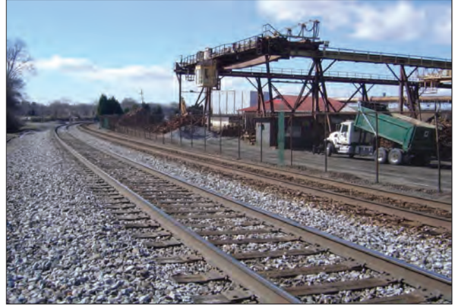
Charlotte Pipe & Foundry - Various addresses
