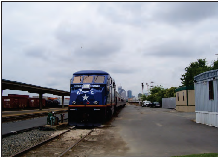
Photo 1 - Existing Charlotte maintenance facility
