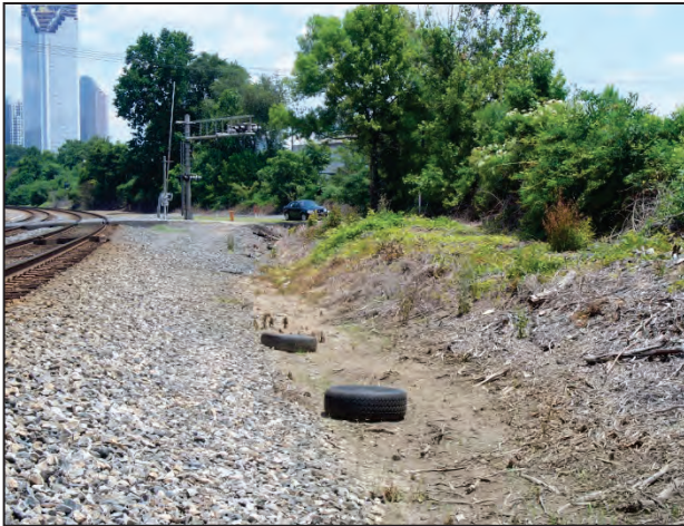
Photo 4 - Existing drainage ditch south of West Summit Avenue crossing
