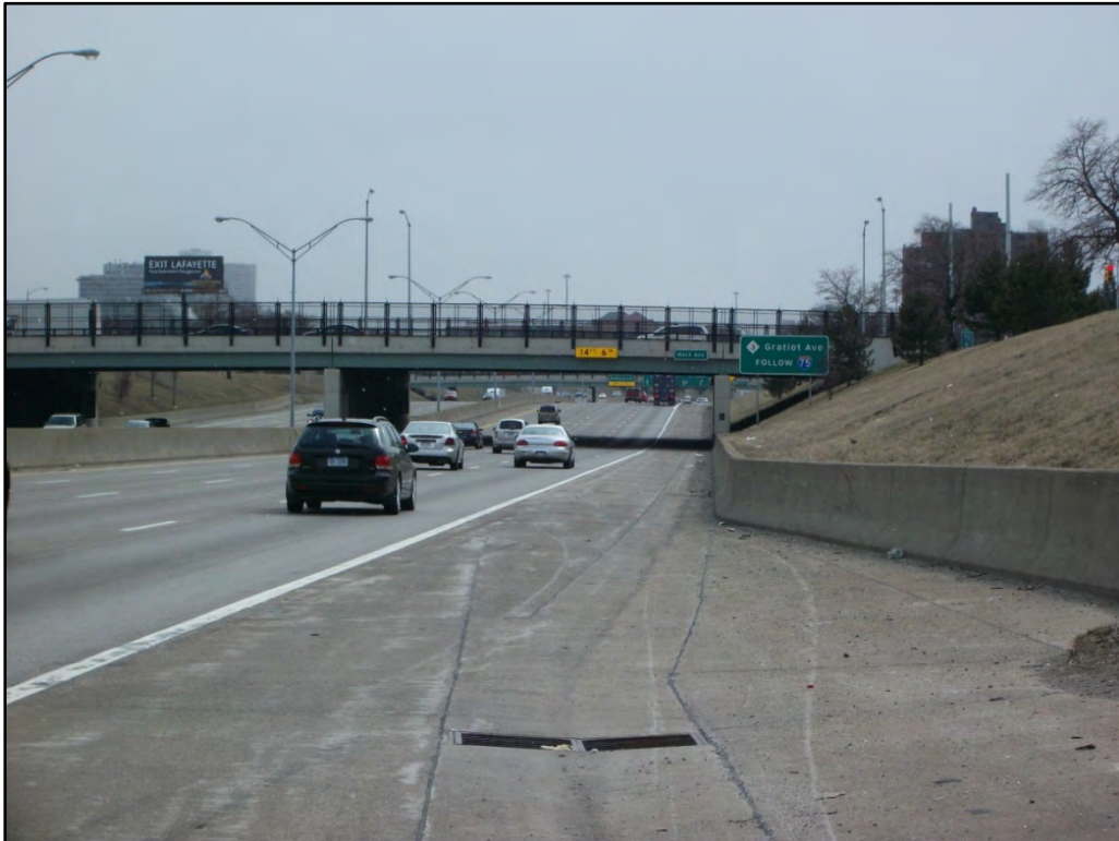
I-75 near Mack Avenue, Detroit, Michigan
