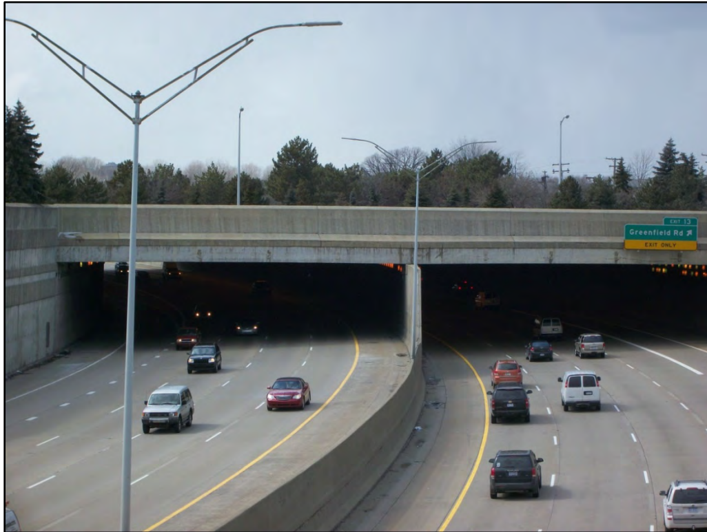
I-696, Royal Oak, Michigan showing a park constructed on top of a bridge over the facility
