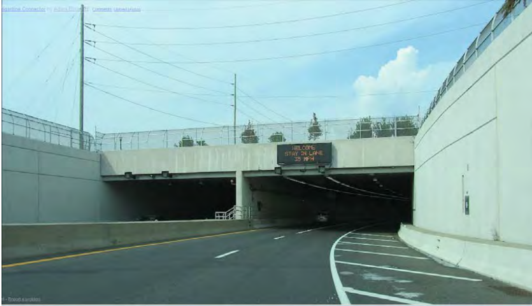
Depressed facility approach to tunnel below water table, Atlantic City, New Jersey
