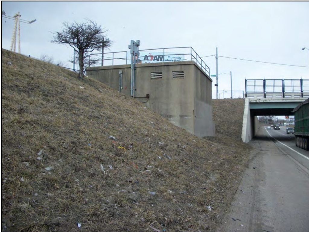
Stormwater Pump Station along I-75 in Detroit, Michigan
