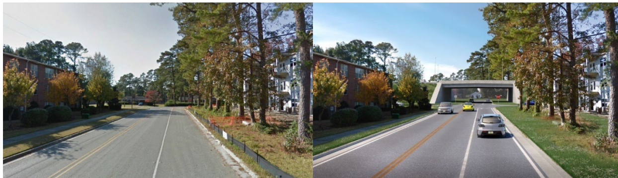
Figure 3-4: View from Darlington Avenue looking west towards Covil Avenue today (left), and with a rendering of the proposed project (right)
