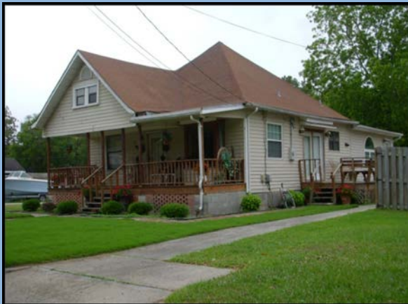
A single-family home located north of Princess Place Drive that is well-maintained.
