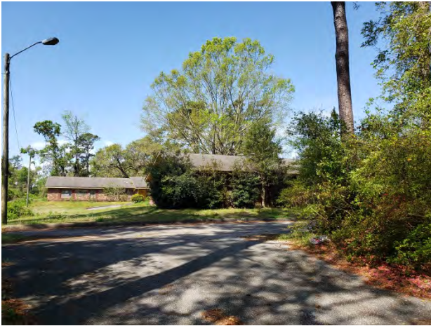
Figure 3: Abandoned apartment complex at 206 Covil Avenue.
