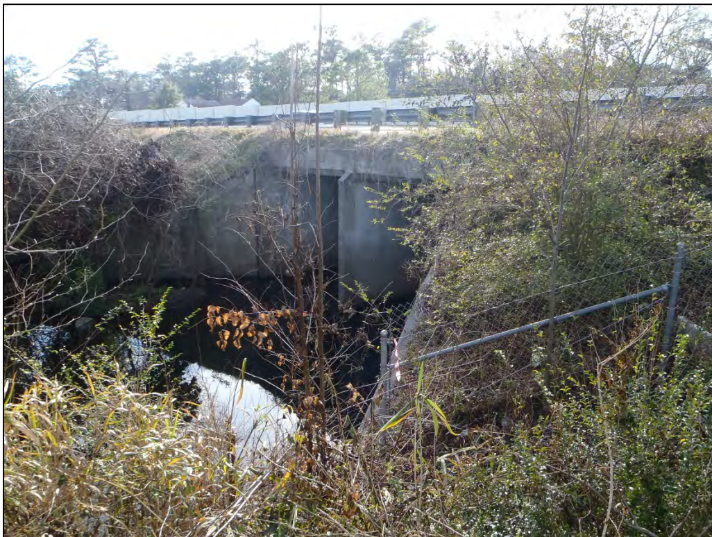
CROSSING 2, DOWNSTREAM (WEST) FACE
