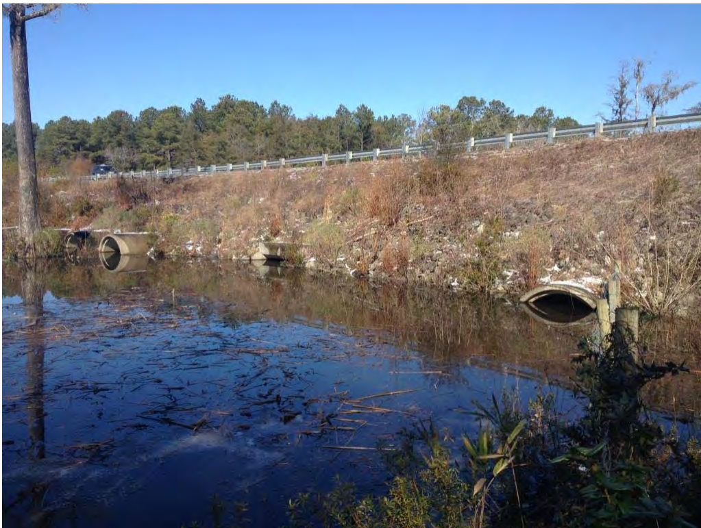
CROSSING 3, UPSTREAM (SOUTH) FACE
