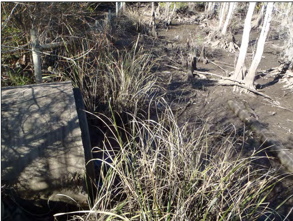
CROSSING 3, DOWNSTREAM END LOOKING EAST
