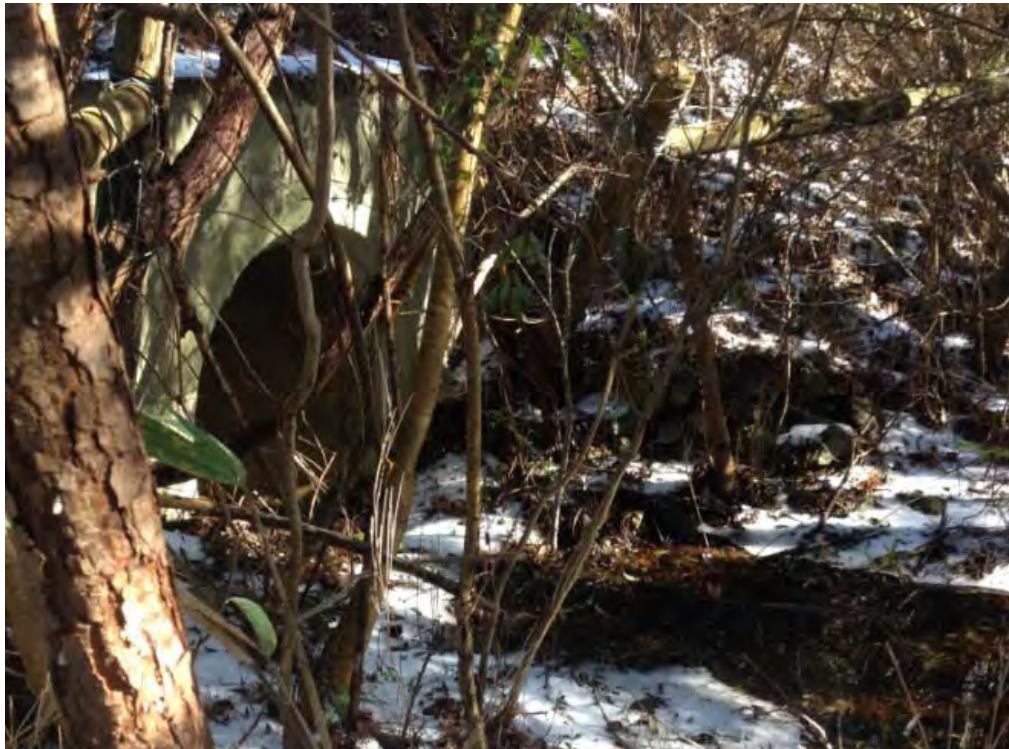
CROSSING 4, UPSTREAM (NORTH) FACE
