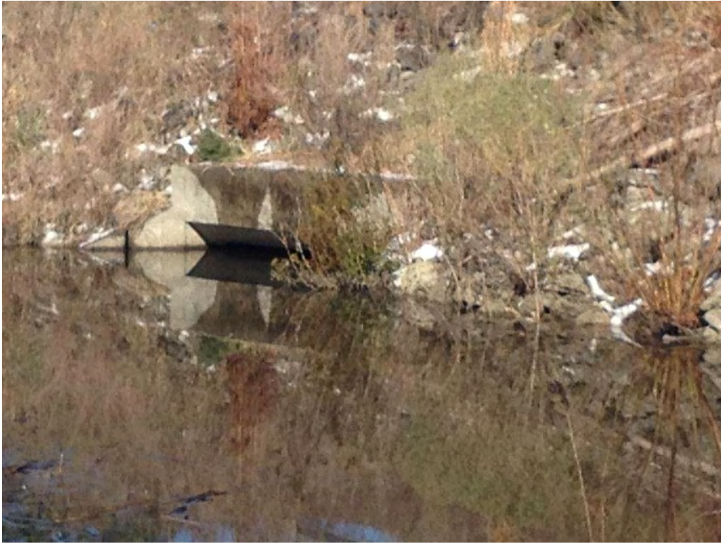
CROSSING 3, UPSTREAM (SOUTH) CULVERT FACE
