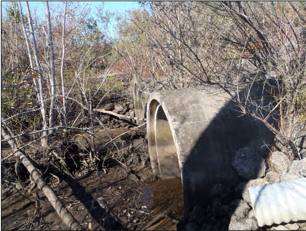
CROSSING 3, UPSTREAM END LOOKING WEST
