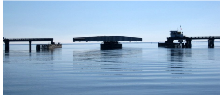
View of the existing Alligator River Bridge with the swing span open for boat traffic NCDOT is proposing to replace the existing swing-span bridge with a modern fixed-span, high-rise bridge on new location.
