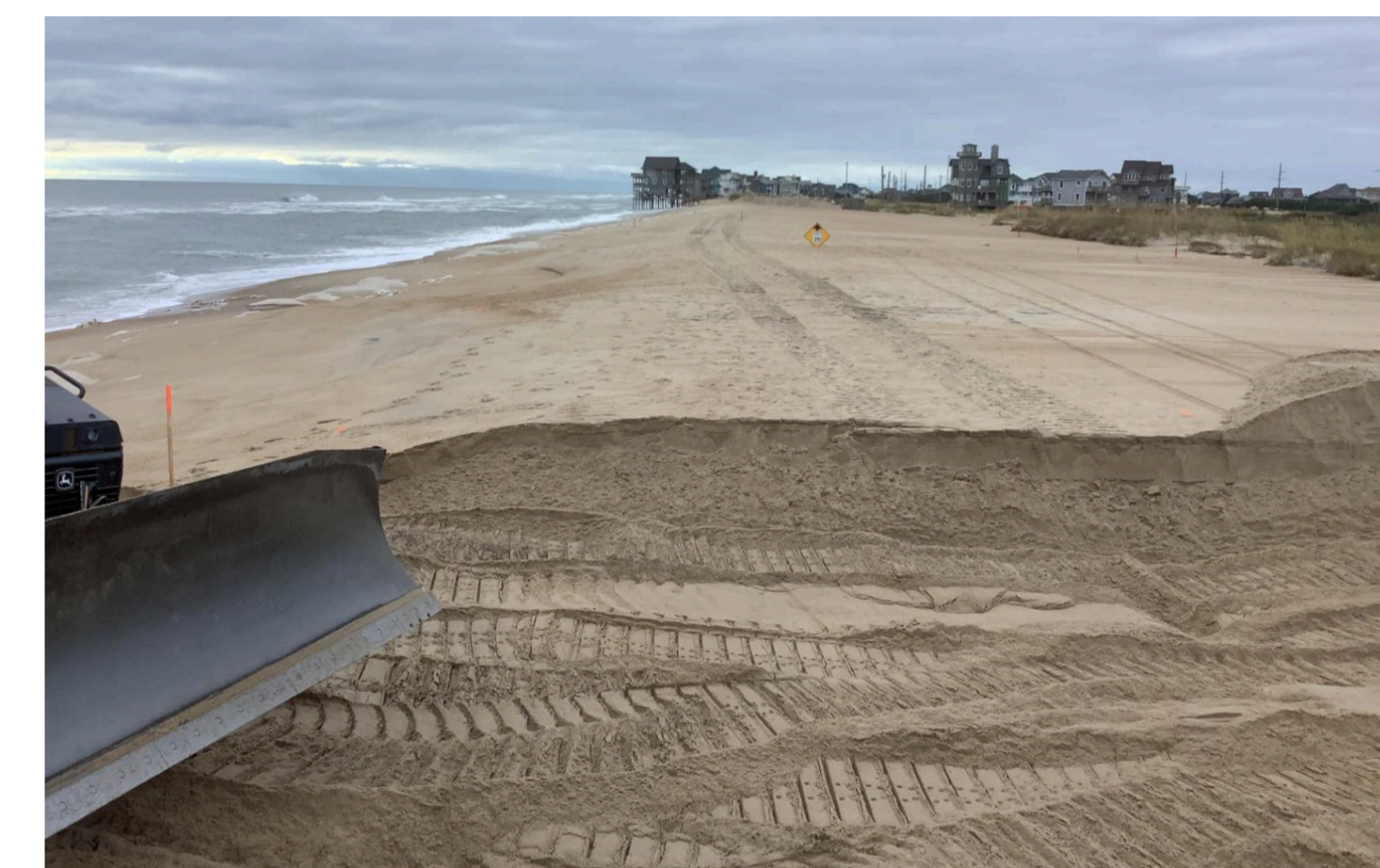
N.C. 12 (invisible under several feet of sand) looking toward Rodanthe after several months without maintenance following construction of the Jug Handle bridge. 2022.
