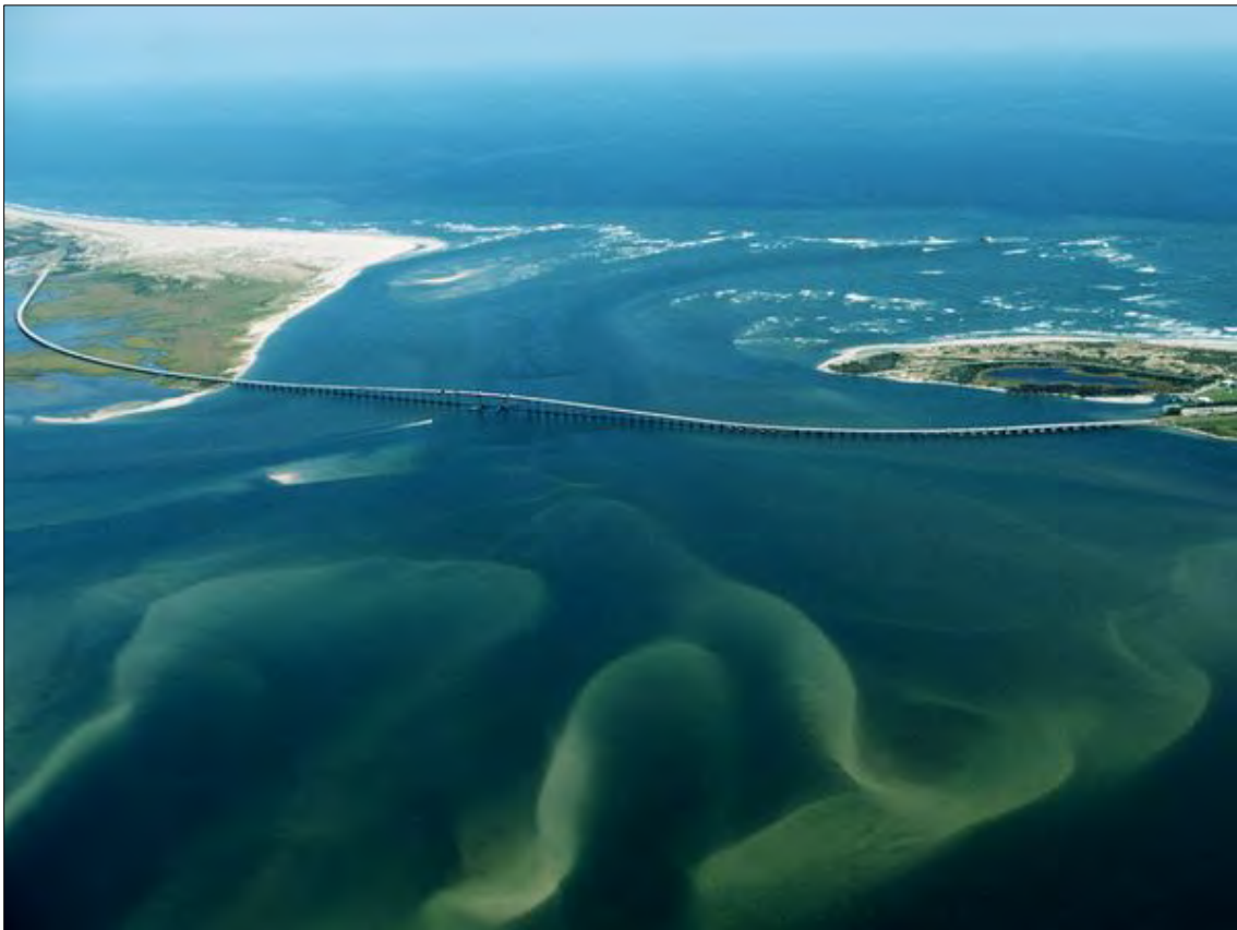
Photo 1. Aerial image of Bonner Bridge.
