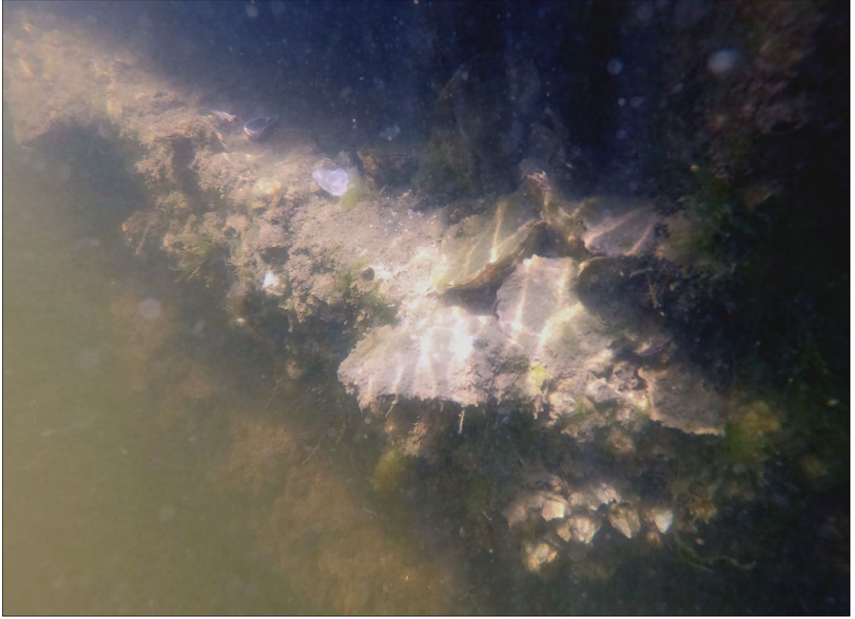
Image III-6. Oysters colonizing a rock on a medium elevation portion of the wavebreak structure.
