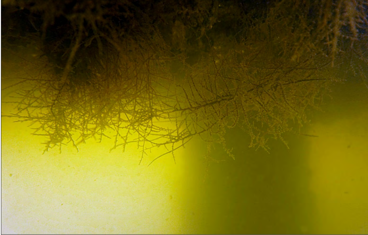
Image III-2. Hydroids colonizing the lower edge of the wavebreak structure. Note support piling in background.
