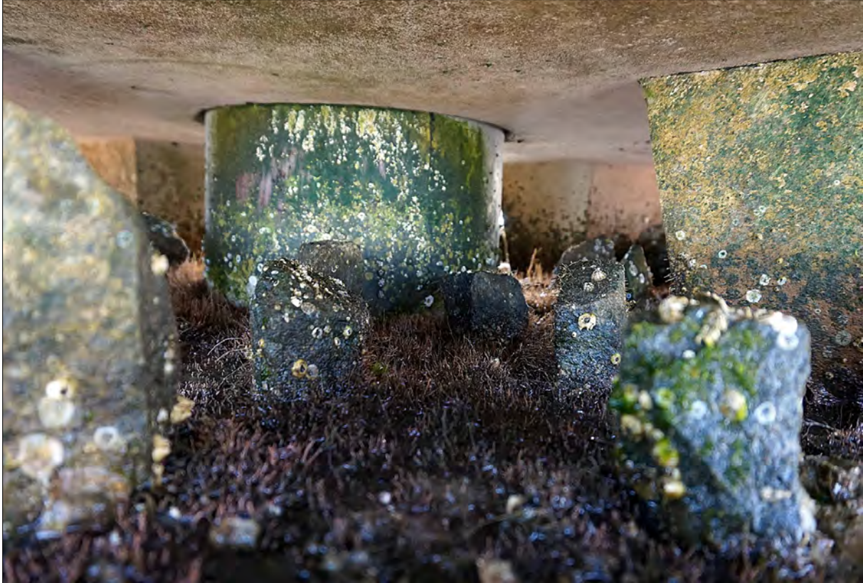
Image III-5. Turf algae colonizing the concrete surface among embedded rocks on a medium elevation portion of the wavebreak structure.
