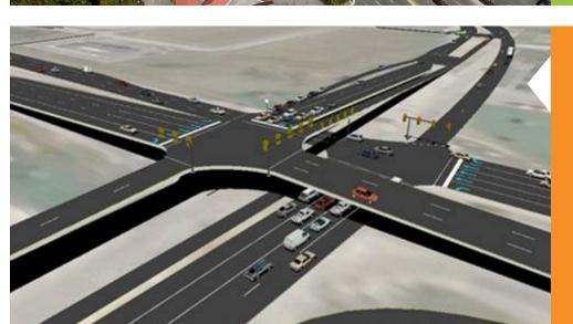
**Echelon Interchange:** This is a computer generated image of an echelon interchange. An echelon interchange places one direction of each of the roads on a bridge, resulting in two signalized intersections. These two signalized intersections can operate very efficiently. Only one such interchange currently exists, in Aventura, FL.
