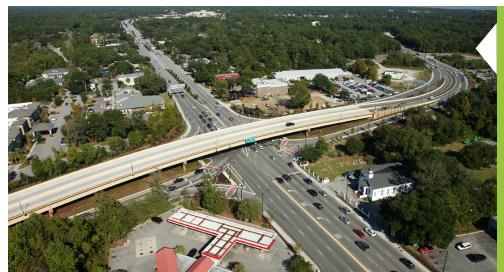
**SPUI:** This example is from Mt. Pleasant, SC. A single-point urban interchange separates the through Ramps will accommodate turning traffic. With the ramps placed very close to the bridge as shown in the example, a single-point urban interchange can be built without taking up much more land than a conventional intersection.
