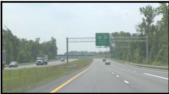
US 264 east of I-95 (Wilson Bypass)
