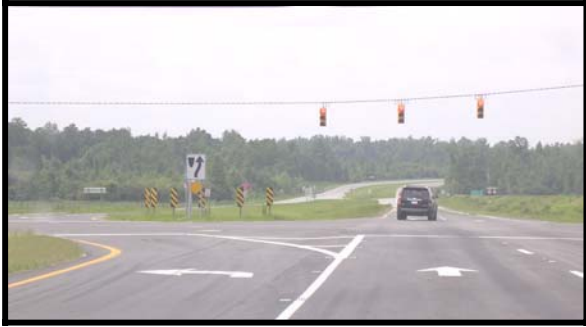
NC 11 (Kenansville Bypass)
