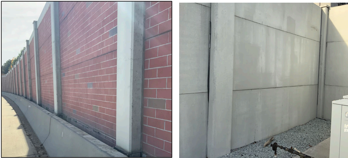
Figure 4: Retaining Walls and Sound Barrier Walls Inspection Results Sample
