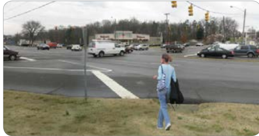
▲ Example of NCDOT-owned and maintained roadways in Belmont, NC, with low LOS for pedestrians.
