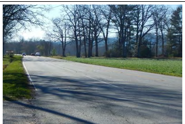
Looking east along NC 191 (Haywood Road) at the SR 1314 (Ladson Road) intersection
