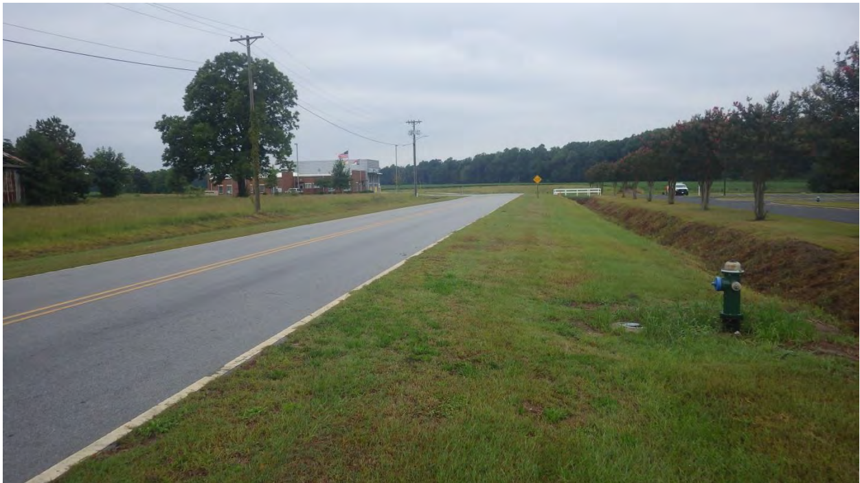
Figure 15. Area 5 Carey Road (SR1571) Overview of Disturbances, View Northwest.
