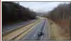
Looking west from Liberty Road overpass.
