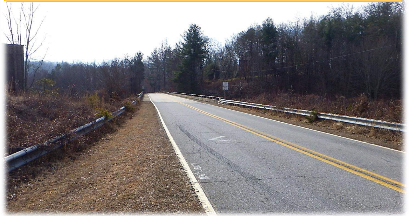
Liberty Road overpass, looking south
