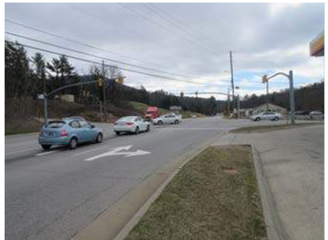
Figure 6: Northern terminus, Sweeten Creek Road at Rock Hill Road, facing south
