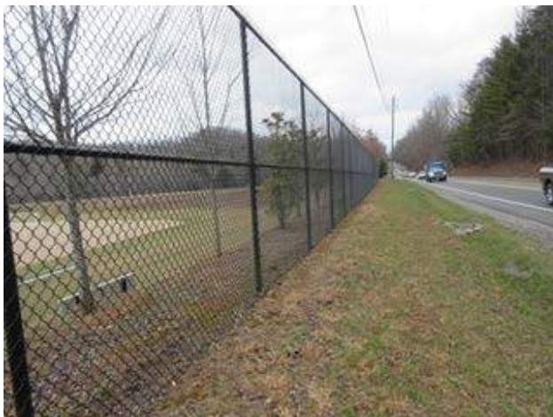
Figure 5: Fencing for Carolina Day School Athletic Complex, on Sweeten Creek Road, facing north
