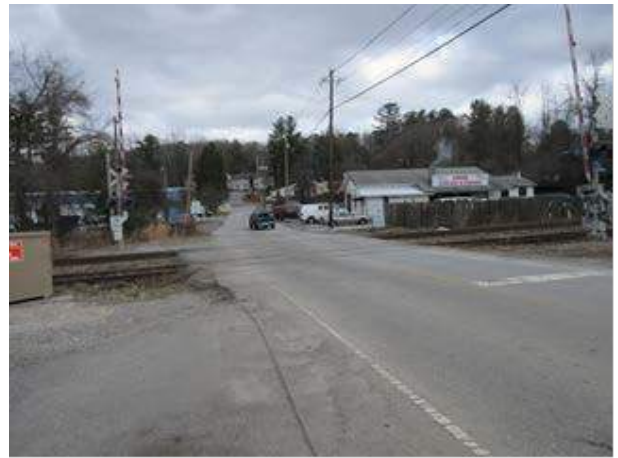
Figure 10: Buck Shoals Road railroad crossing, west of Sweeten Creek Road, facing east
